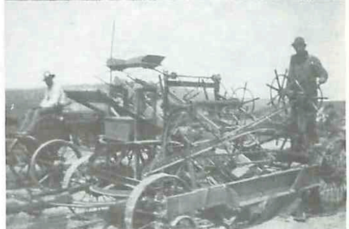
Grading country roads
